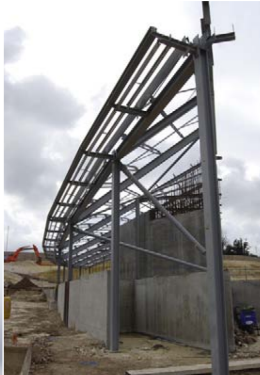
The North Stand, which will accommodate away supporters, takes shape
